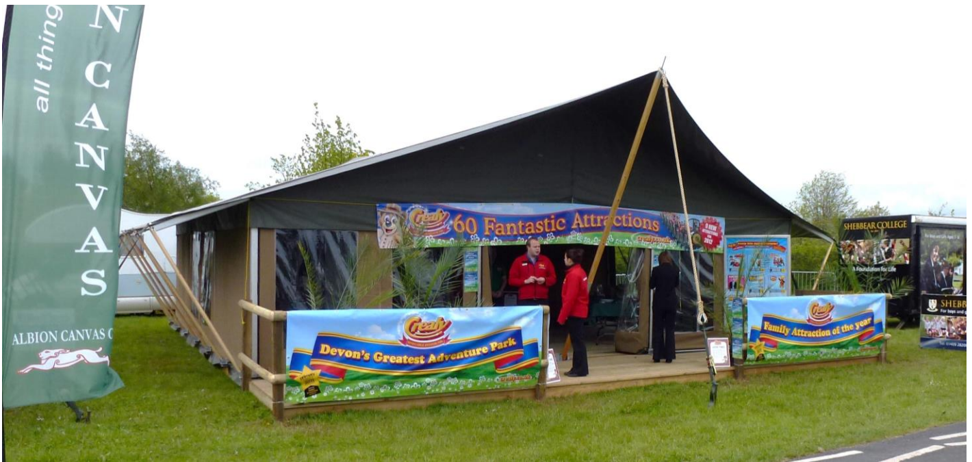
Standard 9m x 9m clubhouse showing guy ropes and side poles.
